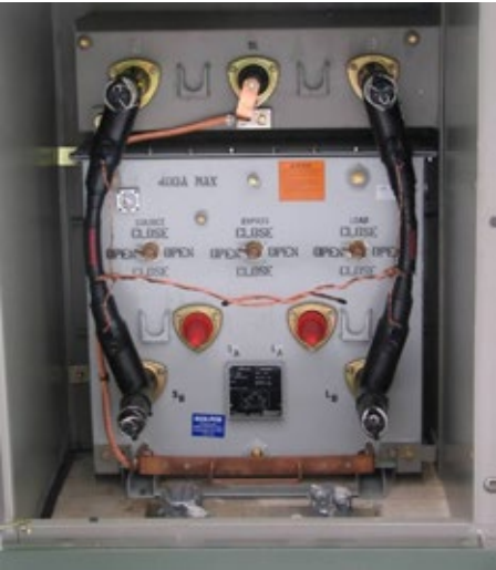
Figure 7. Voltage regulator bypassing operation.
